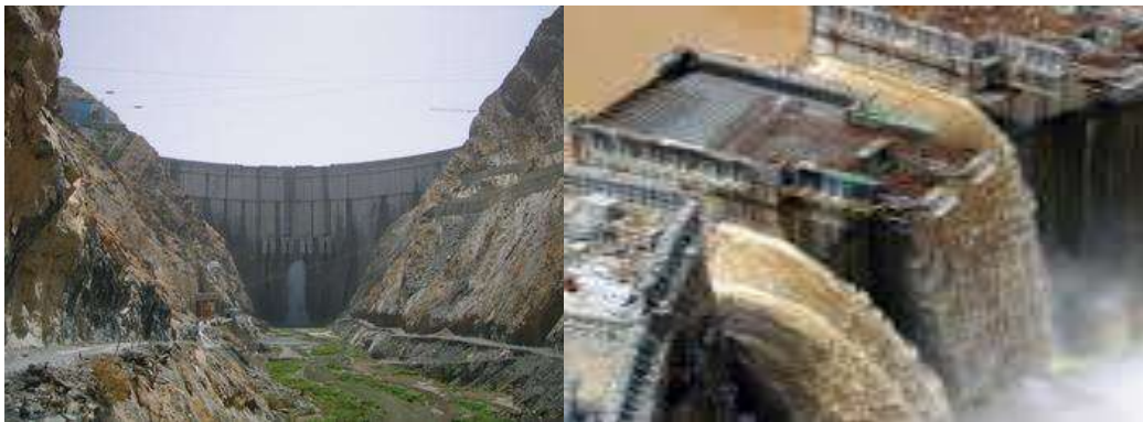
Fig.3 Constructed Hydropower Dam (Tekeze Arch Dam)
