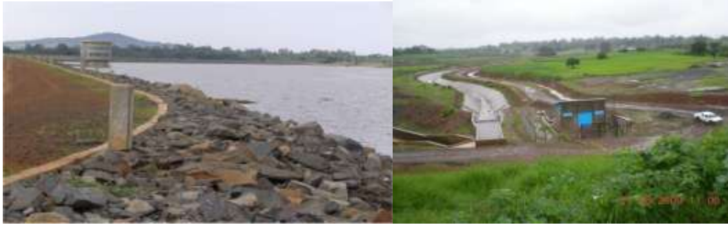
Fig . Current Irrigation Development Project (koga)
