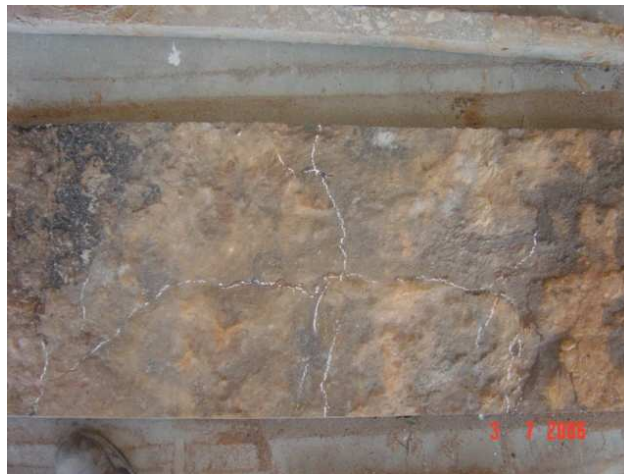
FIGURE 10c View of underside of HMA extracted from full scale test section 4 for diagnostic investigation showing marked positions of cracks.
